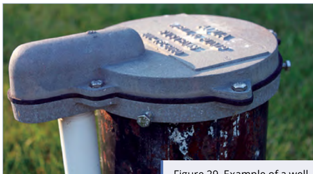
Figure 29. Example of a well cap made of aluminum.
