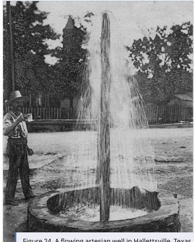
Figure 24. A flowing artesian well in Hallettsville, Texas. Source: Fey and Brautig, Artesian Well, Photograph, n.d.; digital images, ( texashistory.unt.edu/ark:/67531/metaph128796/m1/1/ ), University of North Texas Libraries, The Portal to Texas History, texashistory.unt.edu ; crediting French Simpson Memorial Library, Hallettsville, Texas.
