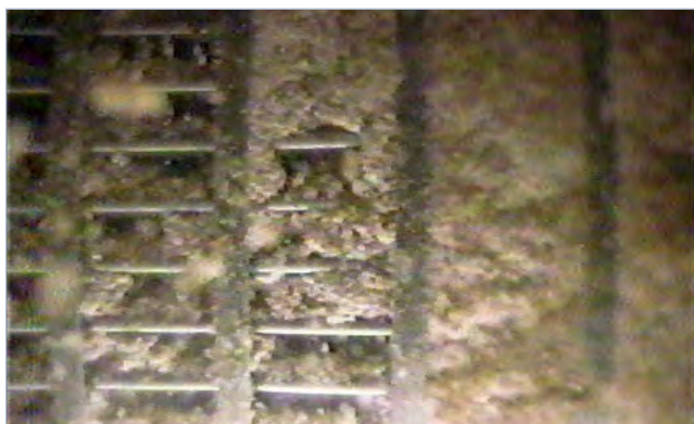
Figure 39. Scale formation on a well screen. (Source: Gary Hix)
