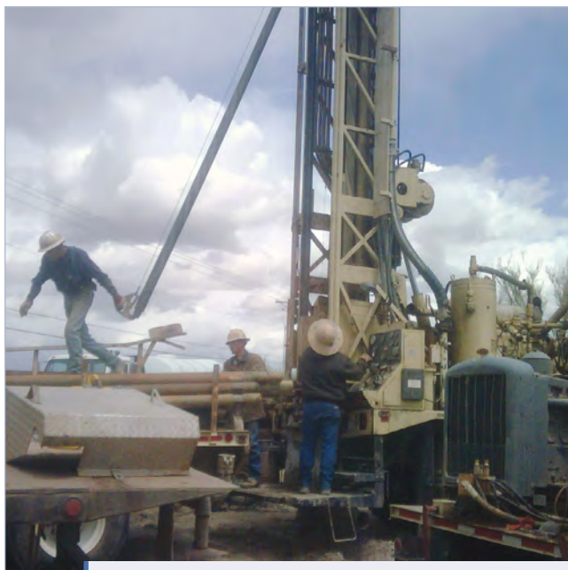
Figure 37. Drilling and installing a well. (Source: Gary Hix)
