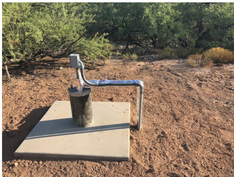
Well plumbing insulated
