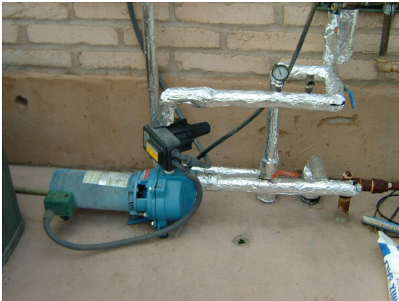
Booster pump insulation
