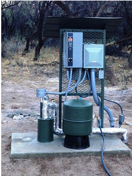
Above ground well insulation
