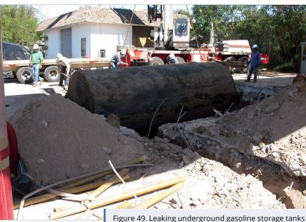
Figure 49. Leaking underground gasoline storage tanks are a common source of groundwater contamination.
