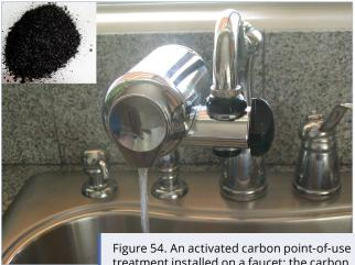
Figure 54. An activated carbon point-of-use treatment installed on a faucet; the carbon media is shown in the photo insert.
