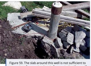
Figure 59. The slab around this well is not sufficient to prevent surface contaminants from entering the aquifer. (Source: *Plugging Abandoned Water Wells*, Bruce Lesikar and Justin Mechell, 2010.)
