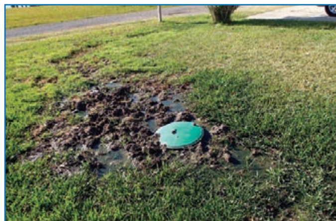
Figure 2. Surfacing effluent around a failing septic tank. Excessive vegetation, foul odors, stained soils, and saturated ground can indicate that the septic system is failing.
